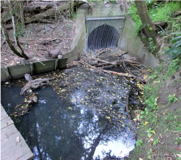
Stormwater outlet Panmure Basin - photo Munroe Graham
